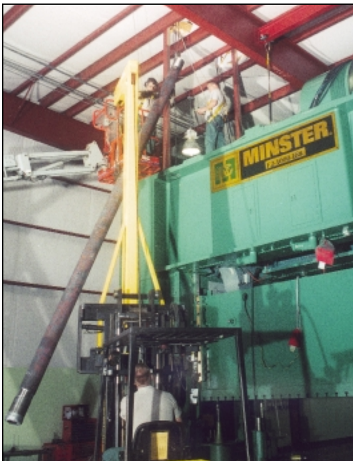
Tie rod is hoisted through a hole cut in the roof.
