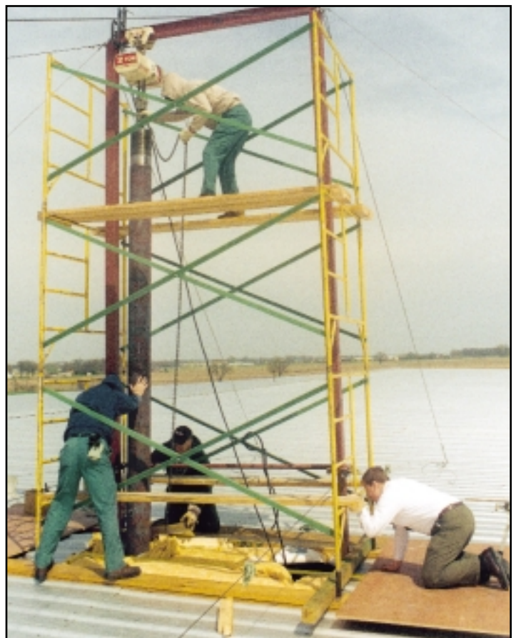
Bryan Pax (right) inspects as tie rod is lowered into press by maintenance personnel at Pax.
