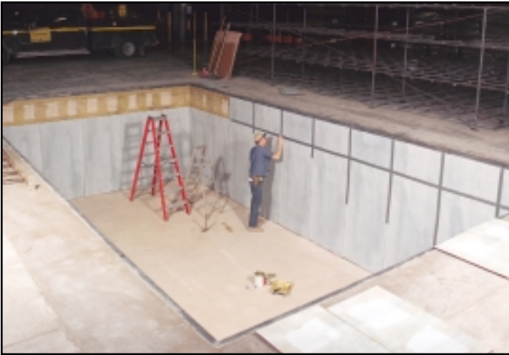
The Pax Lubrication System begins with the press foundation. Once the pit is ready, a layer of anti-vibration material is applied. This helps reduce the vibration throughout the press room.
