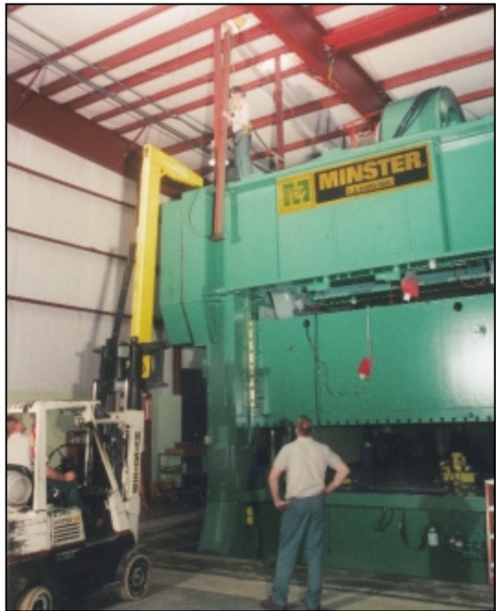
Supports for roof-top crane constructed on top of press.
