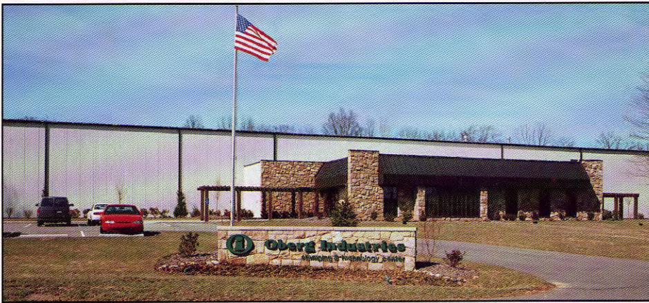
The Oberg Industries Stamping and Technology Center opened in 1994 near the company's headquarters in Freeport, P.A.
